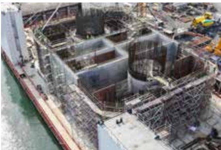
For the offshore wind farm Kriegers Flak, in Denmark, Jan De Nul Group designed and built the concrete foundations for the offshore electrical substations, on a floating pontoon. We were also responsible for transporting and installation.
