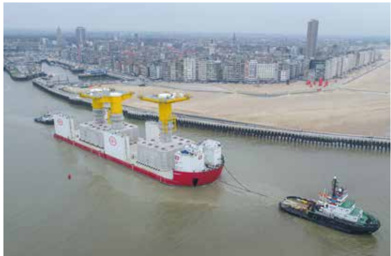
For the offshore wind farm Kriegers Flak, in Denmark, Jan De Nul Group designed and built the concrete foundations for the offshore electrical substations, on a floating pontoon. We were also responsible for transporting and installation.
