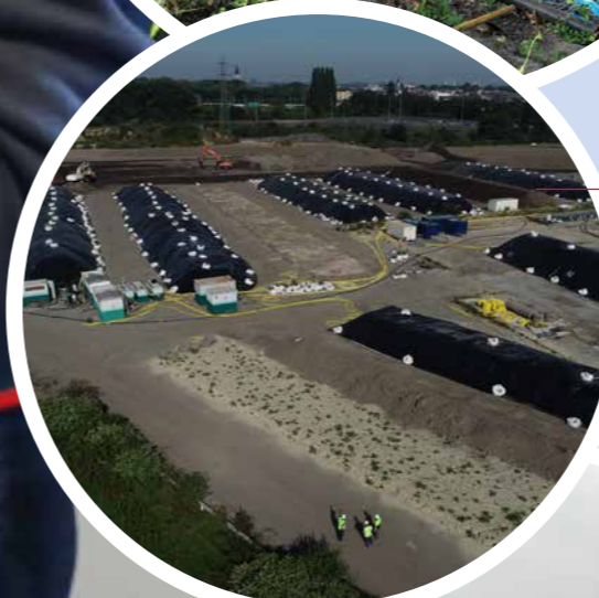
In biopiling, we let nature do its work with micro-organisms.
