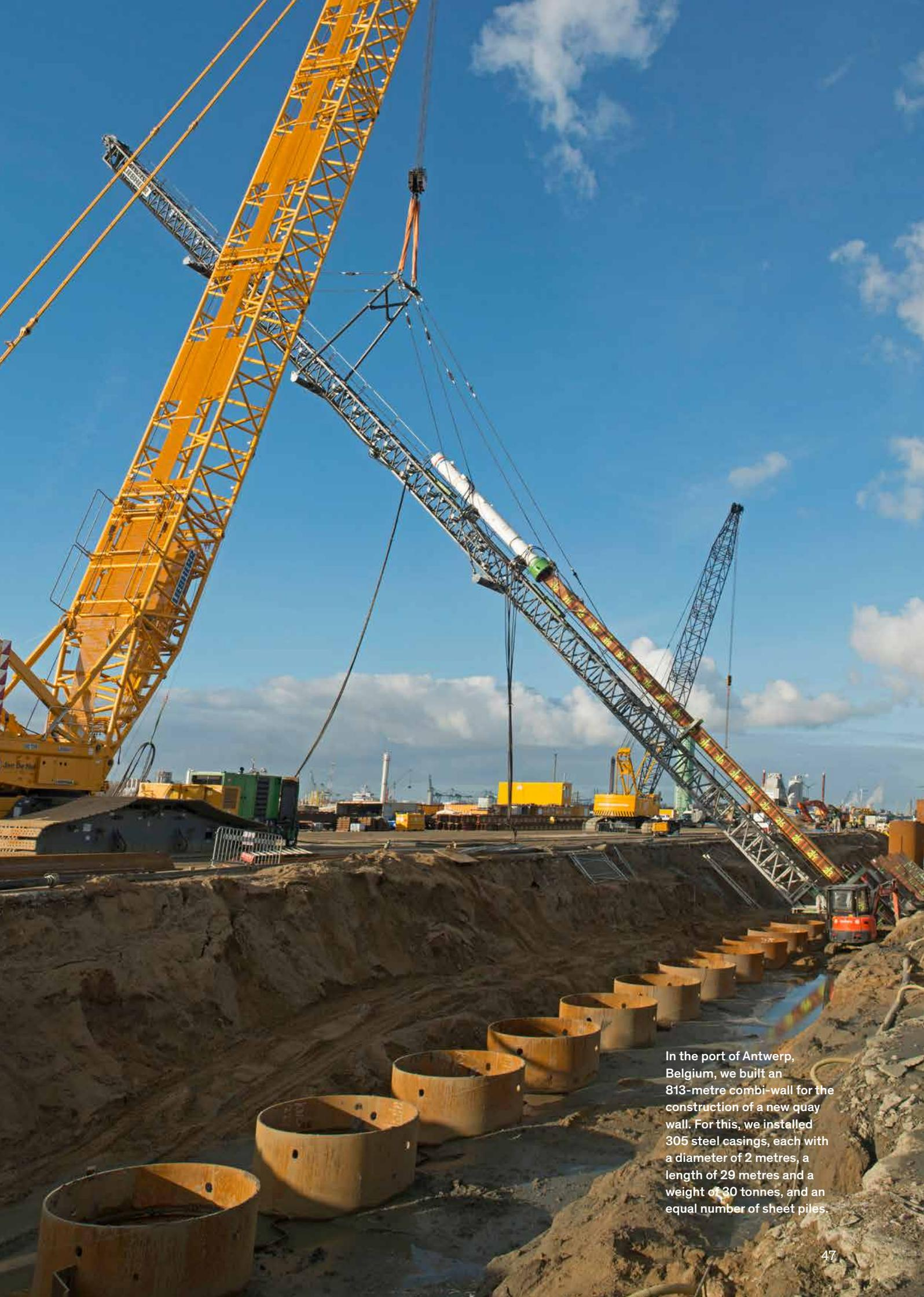
In the port of Antwerp, Belgium, we built an 813-metre combi-wall for the construction of a new quay wall. For this, we installed 305 steel casings, each with a diameter of 2 metres, a length of 29 metres and a weight of 30 tonnes, and an equal number of sheet piles.
