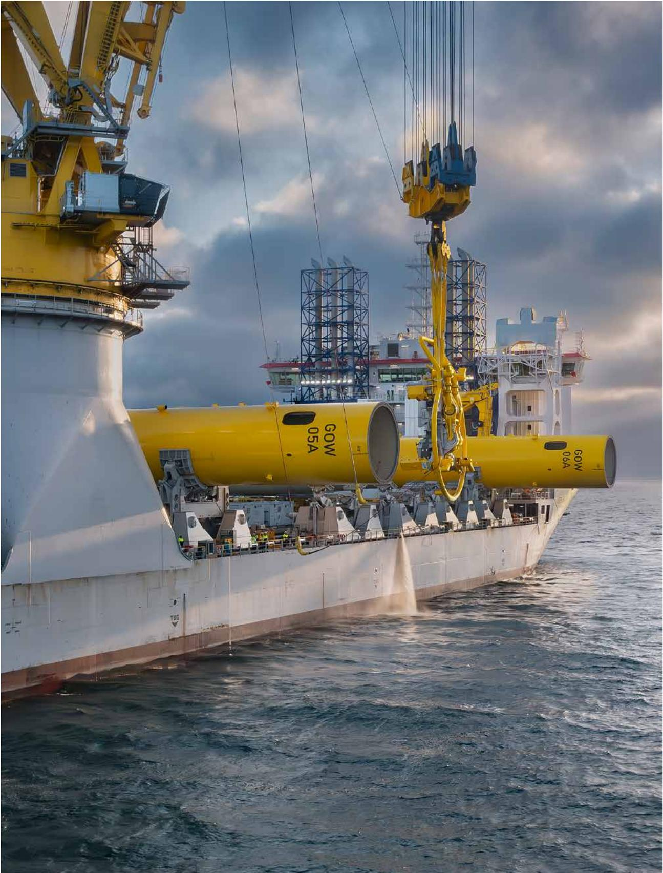
For the German offshore wind farms Gode Wind 3 and Borkum Riffgrund 3, we transported and installed 107 monopile foundations, as well as an offshore substation topside. These wind farms will power 1.2 million German households.
