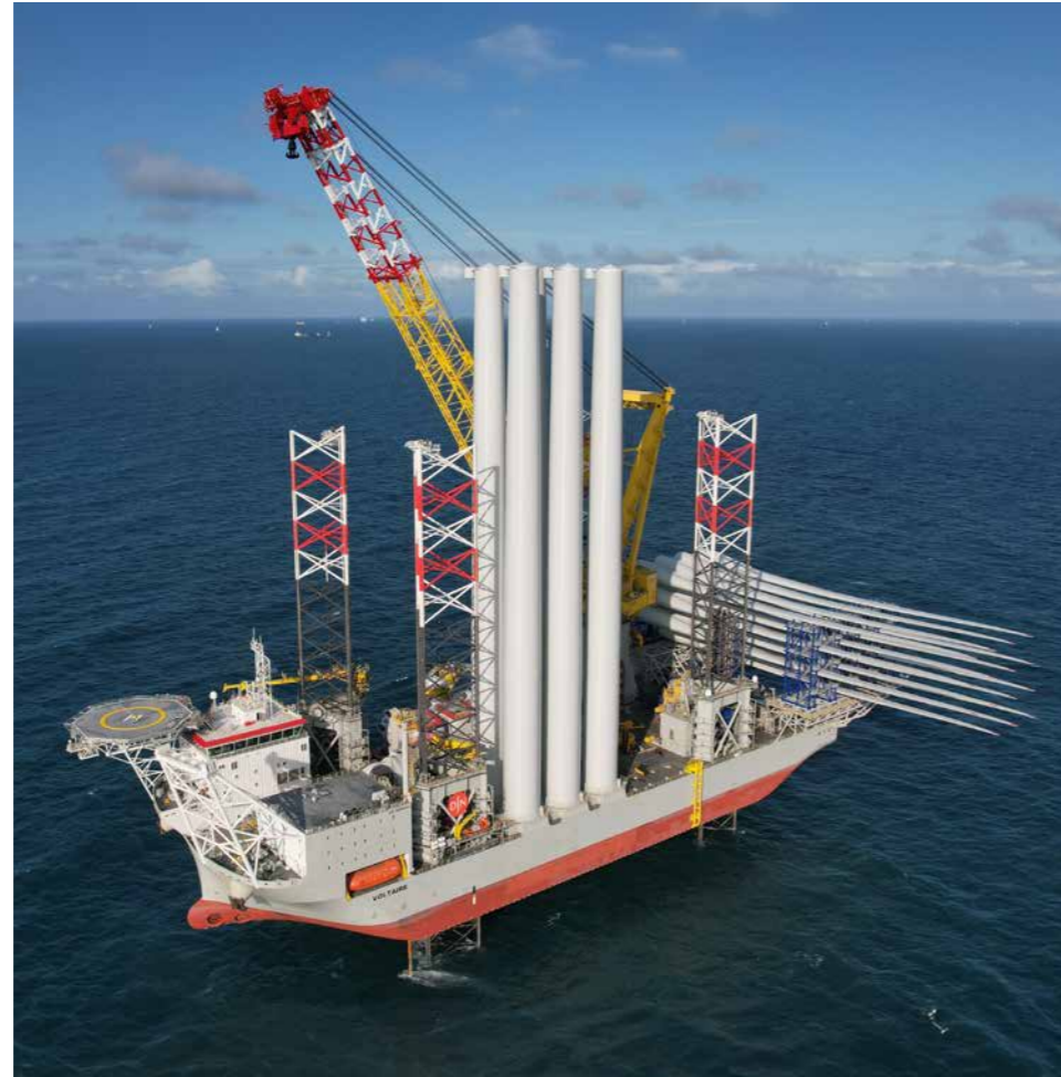
For the offshore wind farm Dogger Bank, UK, we transport and install 277 of the world's most powerful wind turbines, each producing 13 or 14 MW. When completed, Dogger Bank will supply at least 6 million households a year with green power.
